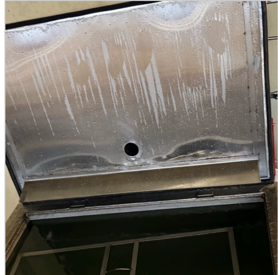
Figure 8. Stainless drip guard flap below the lid edge (lid open). Condensate on the underside of the lid runs onto the flap and back into the tank.
